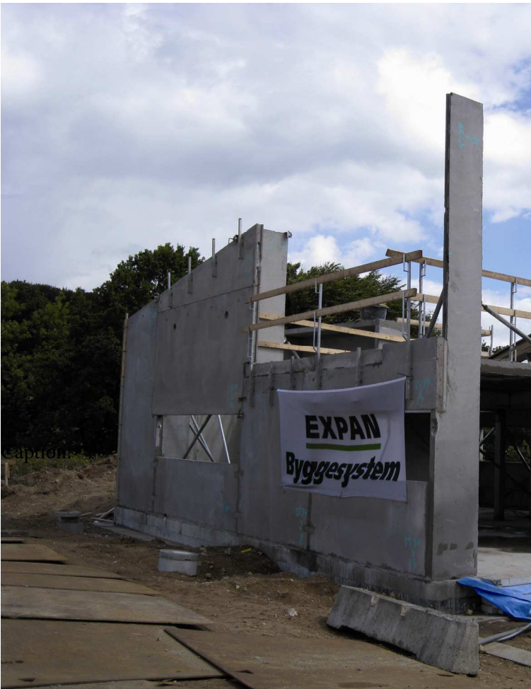
Expan A/S has developed concrete units with fitted ventilation ducts for KOMFORT HUSENE.
